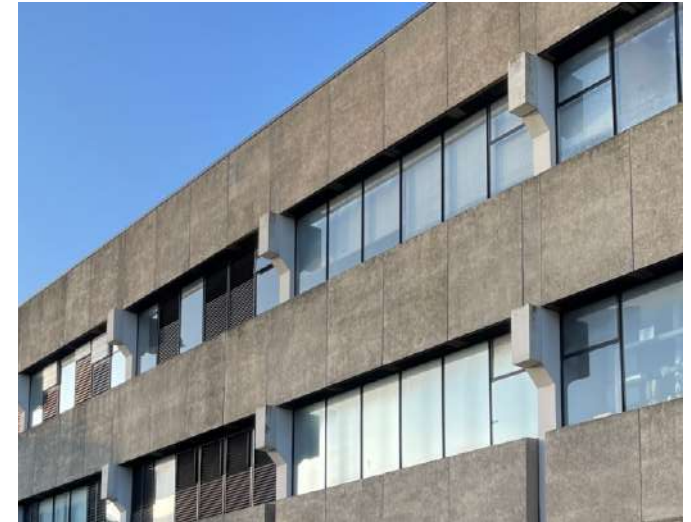
The Telephone Exchange extension. Photo: GCC
