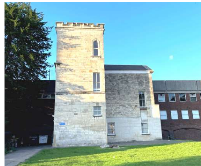
Addison's Folly (Grade II listed) with the Eastgate Shopping Centre visible behind. Photo: GCC.
