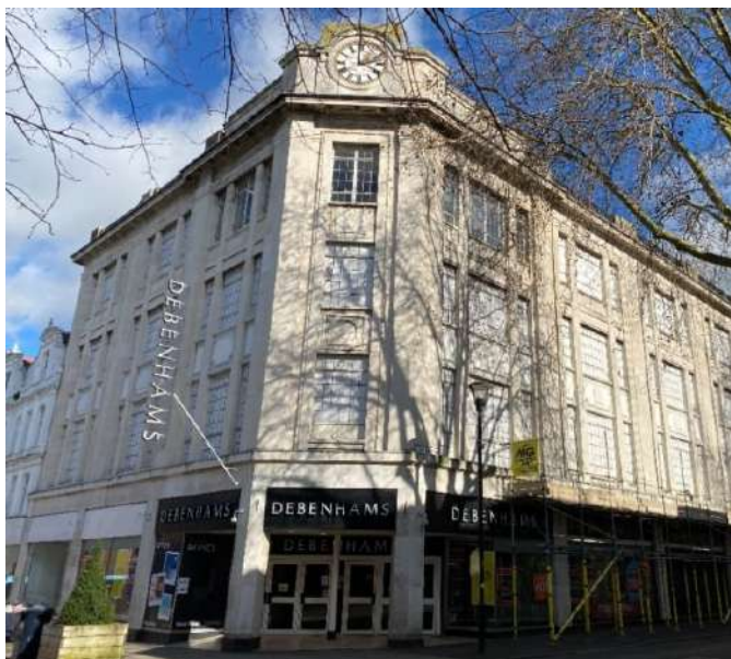
The former Bon Marche/Debenhams building, Northgate Street. Photo: GCC.
