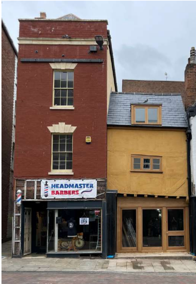
Sixteenth-century timber framing (right) and nineteenth-century brick façade (left) at 39-41 Westgate Street—both Grade II listed buildings. Photo: GCC.
