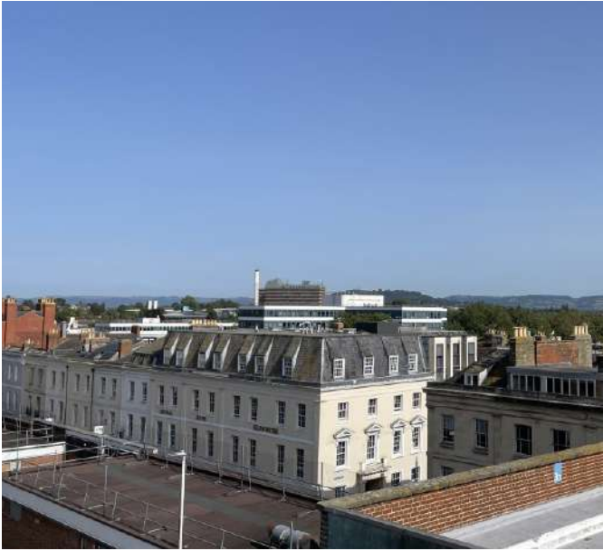
Looking east from King's Walk carpark. Photo: GCC.
