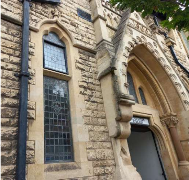
Victorian gothic details on the Public Library, Brunswick Road. Photo: GCC.
