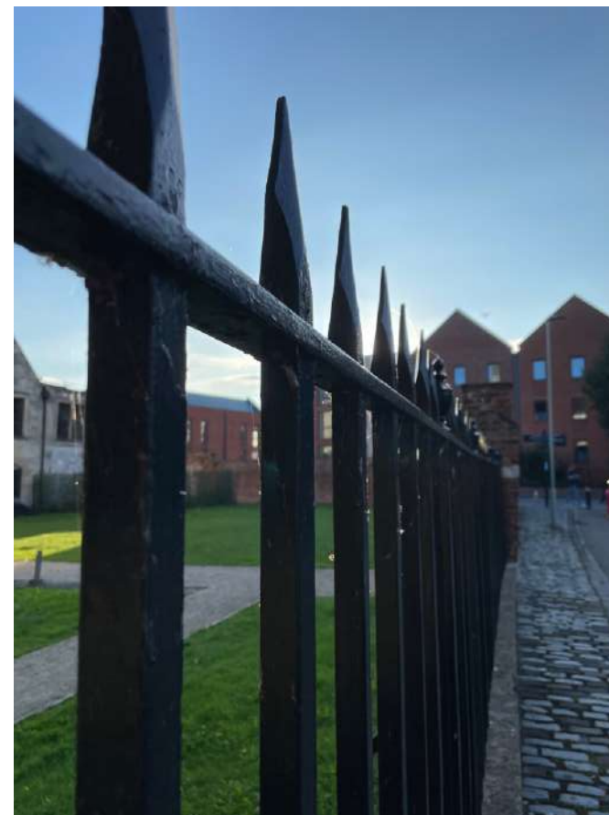
Boundary railings at Blackfriars. Photo: GCC.
